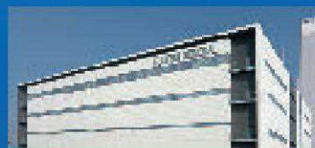
R&D Center (Japan) and 60m height testing tower Central R&D center for global air conditioner development.
