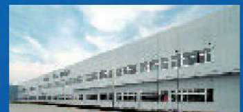
FUJITSU GENERAL CENTRAL AIR-CONDITIONER(WUXI)CO.,LTD. (China) VRF Main factory. ISO9001 and ISO14001 certified.
