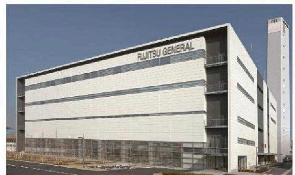
Kawasaki R&D Center and 60m height difference testing tower
