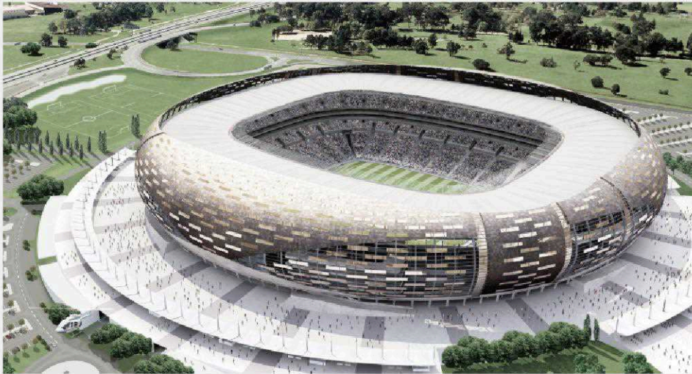
Soccer City – Soccer Stadium of 2010 FIFA Water-cooled Packaged Unit South Africa
