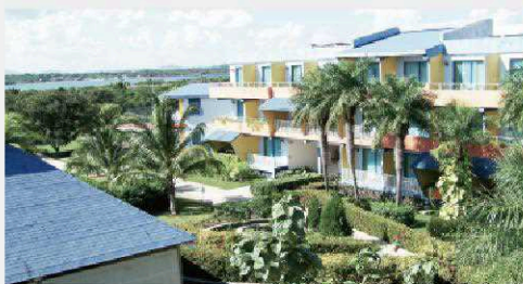
Playa Pesqueto Heat Recovery Air-cooled Screw Chiller Cuba
