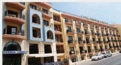
Luna Holiday Complex Water-cooled Screw Chiller Malta
